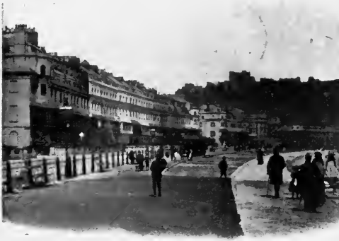
The Parade, Dover. Strong cornice lines on a curve.
